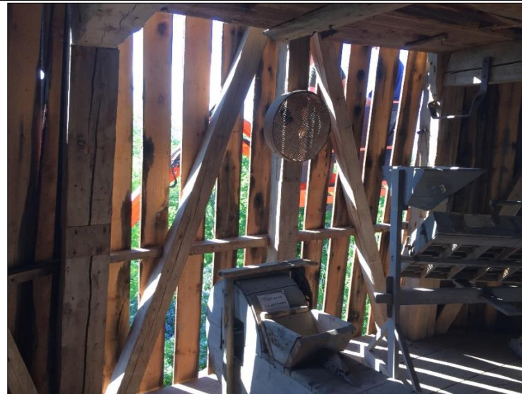
Ny fasadpanel har monterats. Foto: Allan Rodbe, 2020-06-08
