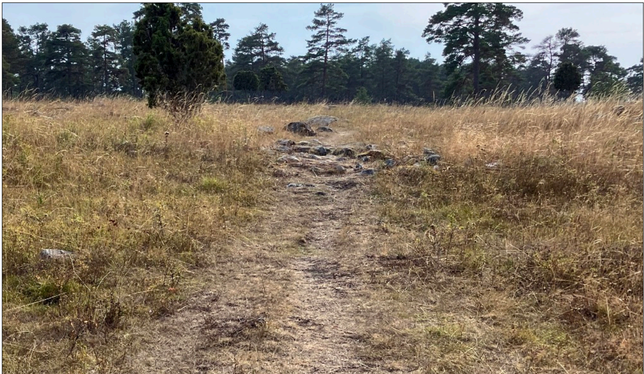
Figure 3. The Eastern part of the embankment seen from the outside. The wall is very low, laying along the terrace and is about 4 meters wide, but only around 0,2 - 0,3 meters high.
